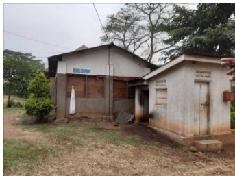
Old building awaiting renovation
